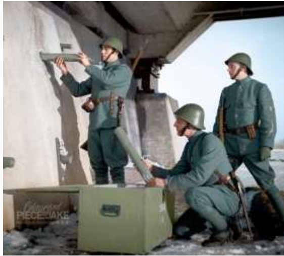
Dutch soldiers place explosive charges in a bridge pillar on the Twente Canal near Goor, Netherlands. In order to delay the German advance the Dutch army blew up several bridges in May, 1940 including this one.
